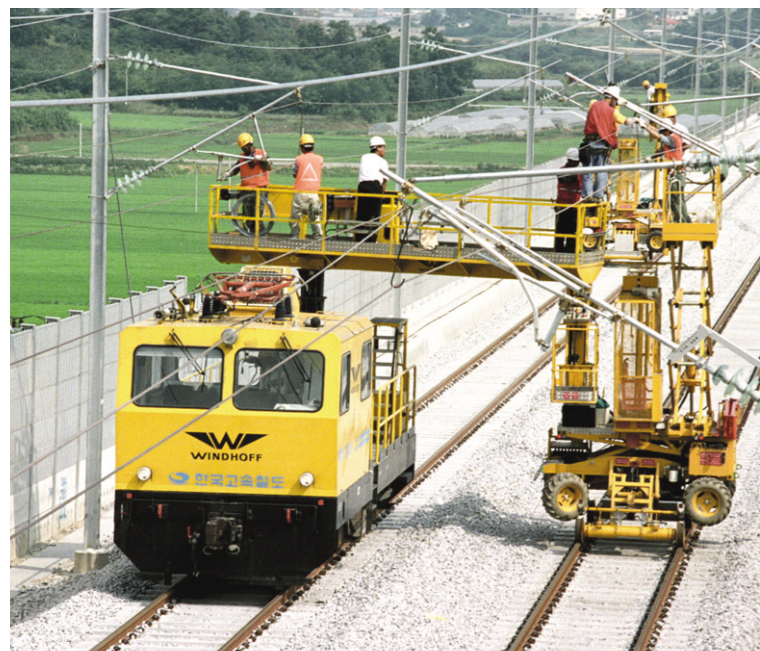
Installation of Catenary
